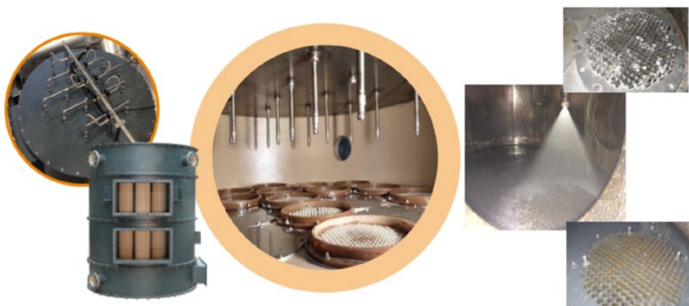
Figure 4: In-line cleaning system for Heat Matrix Polymer Air Preheaters
