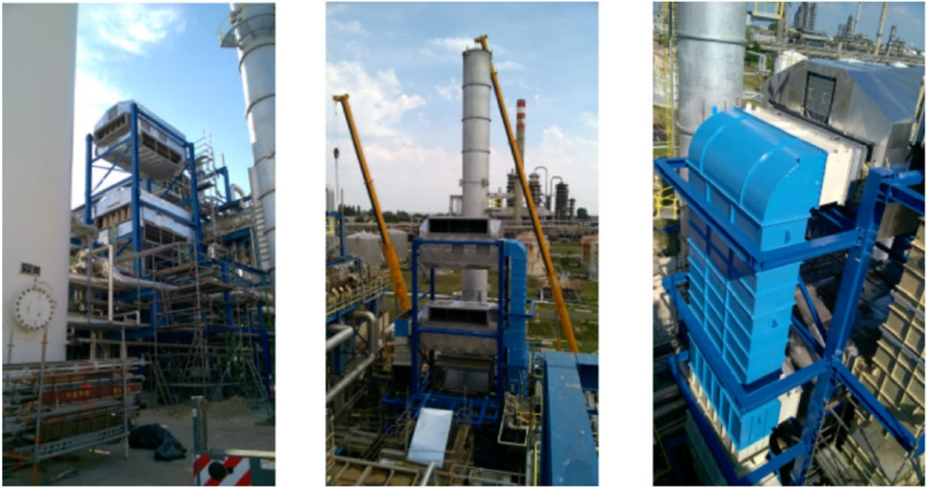
Figure 3: Examples of installed Heat Matrix Air Preheaters
