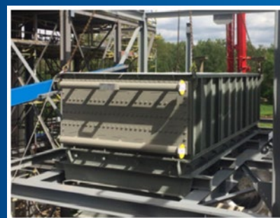
Figure 8: Installed Heat Matrix Polymer ECO
